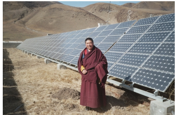
Figure 3: Photovoltaic generator, 40 kW, in front of the new power house in Suohourima
