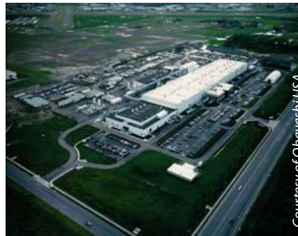
SolarWorld facility in Hillsboro
