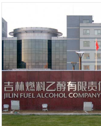
The ethanol plant in Jilin province has a capacity of about 180 MMgy.
