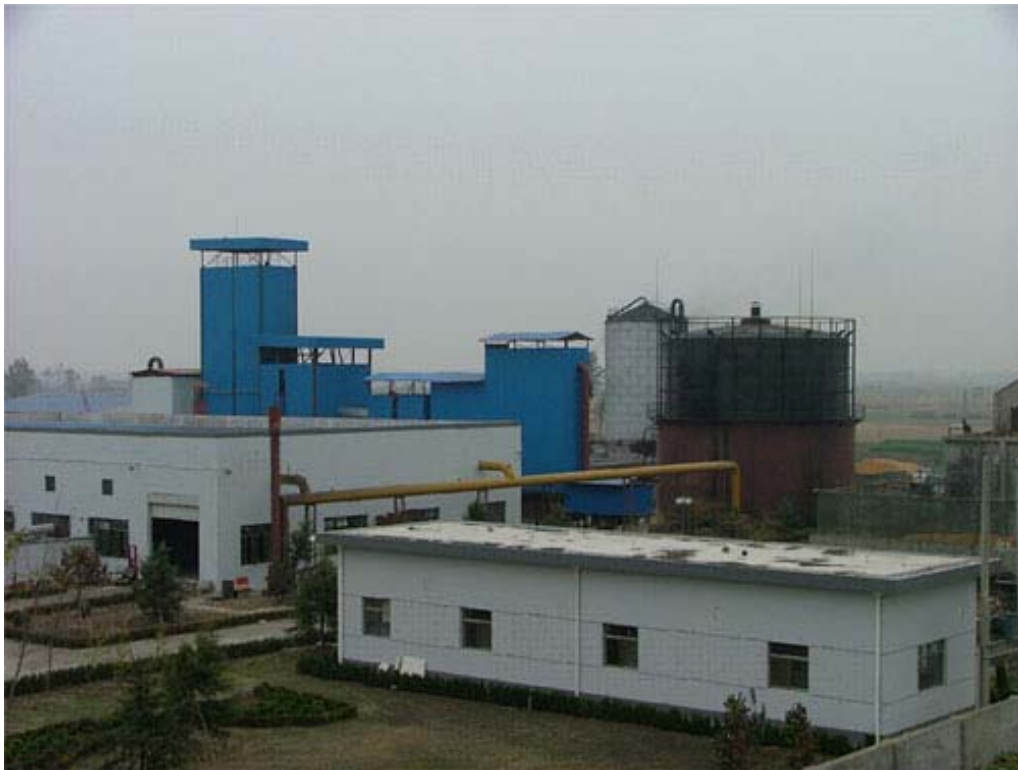
Jiangsu Xinghua Biomass gasification power generation plant
