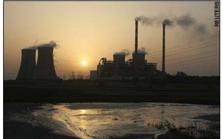
Carbon Capture and Storage could help cut emissions from coal-fired power stations
