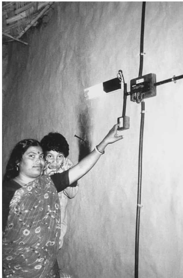
Figure 6. Mother and son try their home lighting system for the first time. (Credit: NREL PIX 05466)
