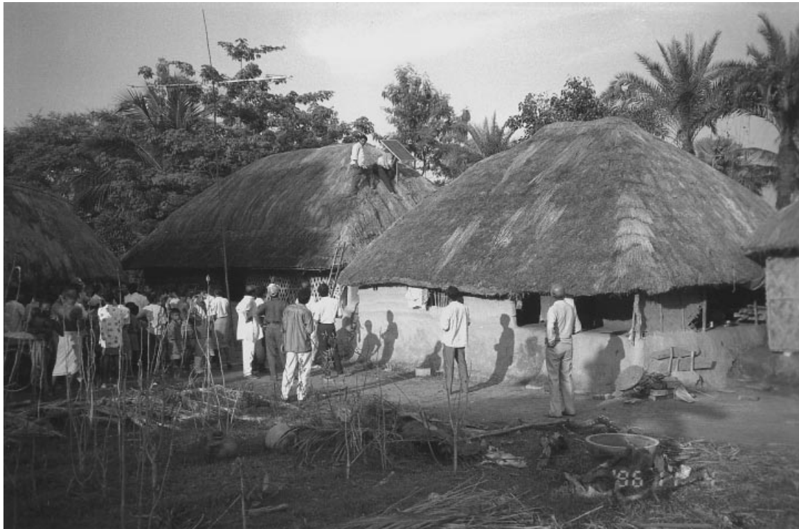
Figure 1. Installation team places a PV module on the home of a village beneficiary. Villagers gather around to witness the event. (Credit: NREL PIX 04877)
