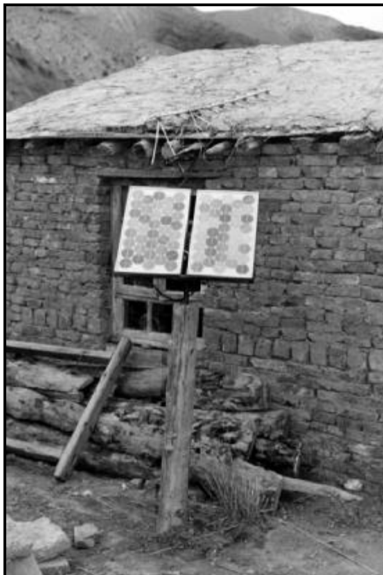
Figure 1. Solar home system installation in Xinjiang Province, typical of such installations in China.
