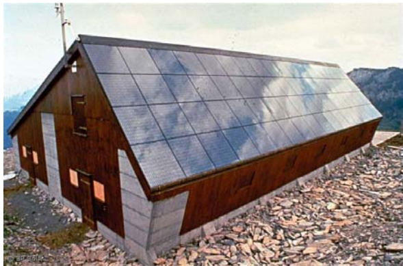
Figure 1.1.5 The sample of BIPV (With the Courtesy of BP Solar)
