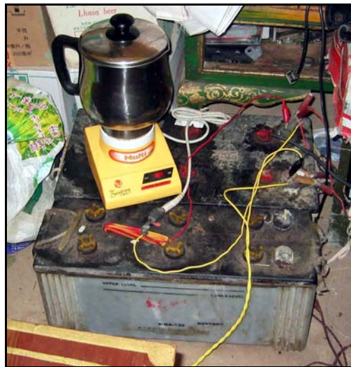
Batteries in a household solar system used to run a hot water kettle.
