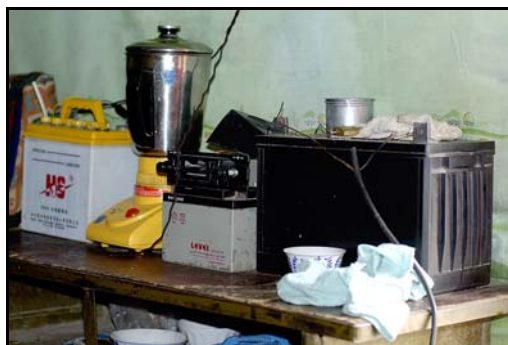
Household appliances powered by batteries charged by PV panels.
