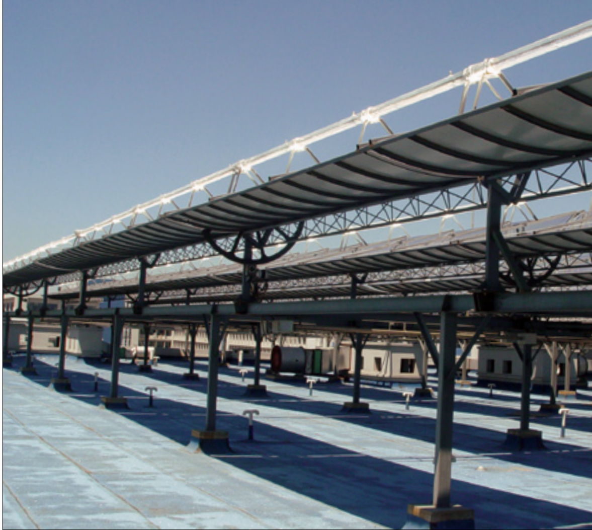
Solar thermal challenge of the future: a system for solar cooling in the town of Tianjin
