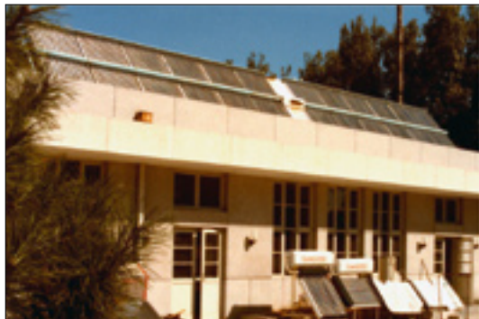
Yin's lab from 1983 to 1988. The first vacuum tubes with the Al-N/Al coating developed by professor Zhiqiang Yin were installed on the »solar house« by the scientists.
