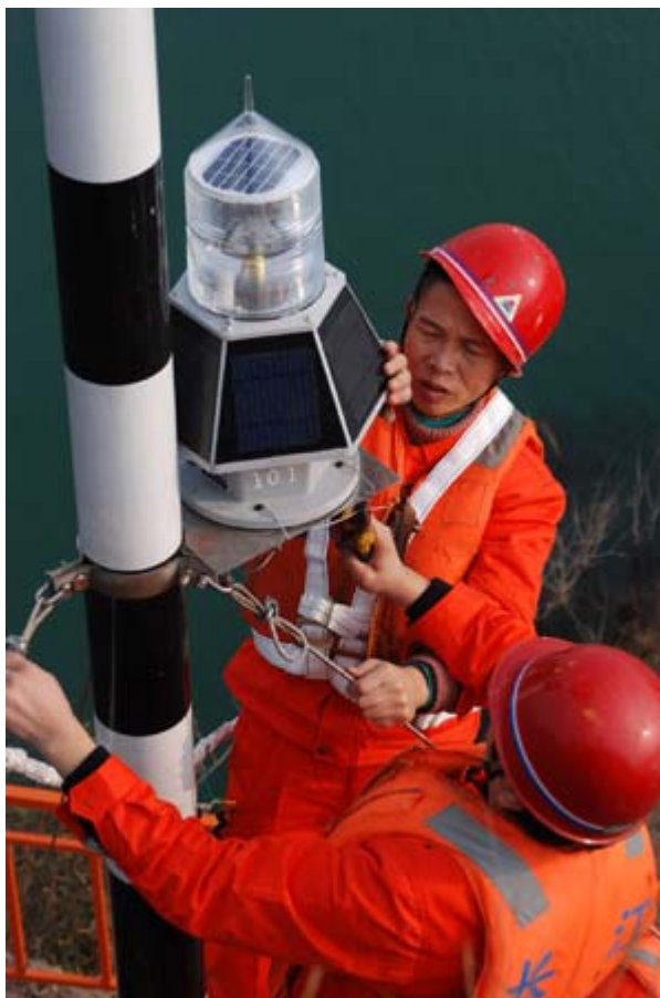
Two workers fix a solar navigating lantern in the Three Gorges area. [China Daily]
