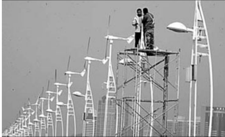
Workers check street lamps powered by wind energy in the Olympic village in Qingdao, Shandong Province, which will host some of the water sports at this summer's Games. [File photo]
