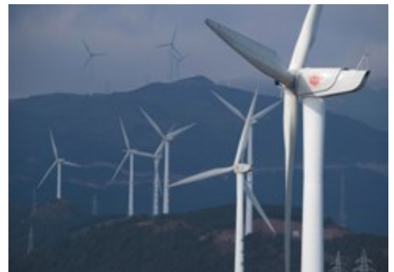
The Dali project, being the highest altitude wind farm in the mainland, comprises 64 wind turbines.
